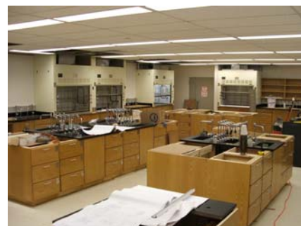
New lab benches and hoods in place; renovation is nearing completion.
