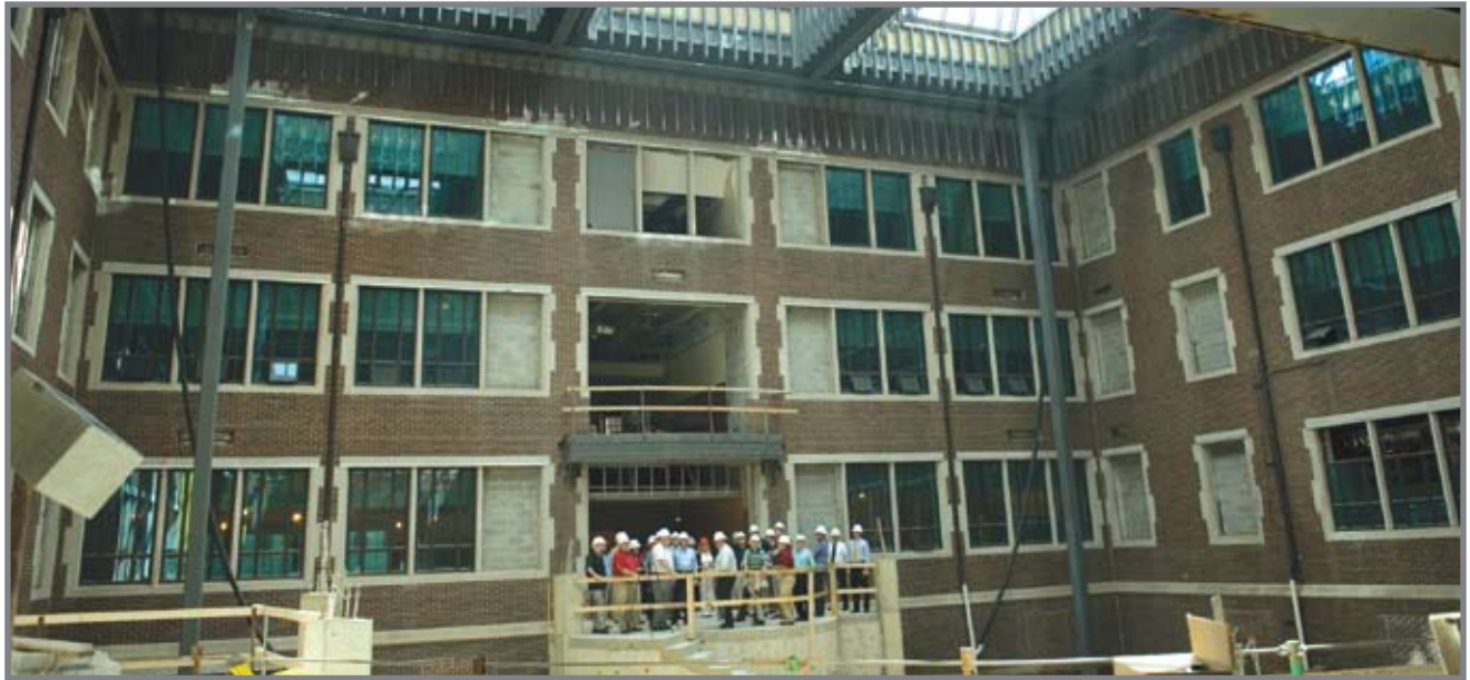
University Hall renovation
